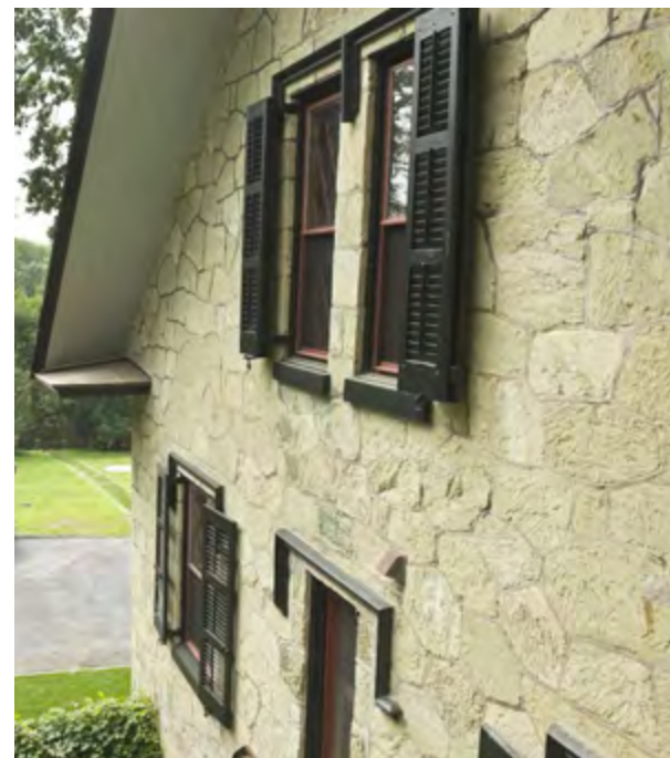
Serpentine is the major building material of Edgewood. Note the greenish hue.
