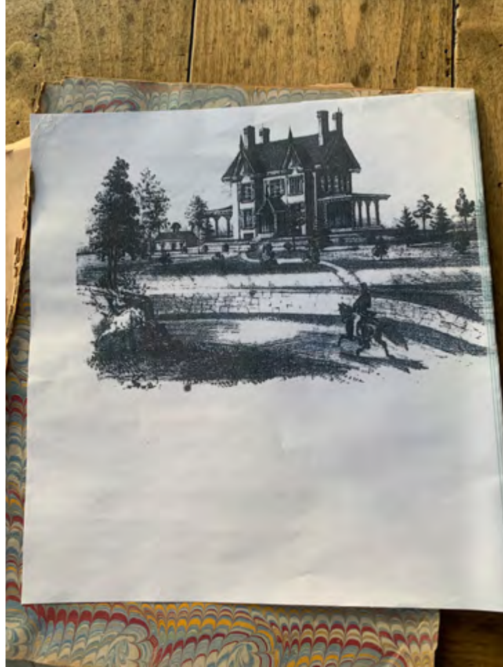
A sketch of the original house, before the tower was added to the left side.
